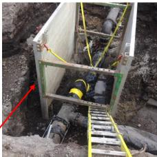
This trench box is in place to protect our employees. We use a ladder placed directly into the confines of the trench box so as not to expose our employees to additional hazards. Note the benched sides of the trench in addition to the added protection afforded by the trench box.
